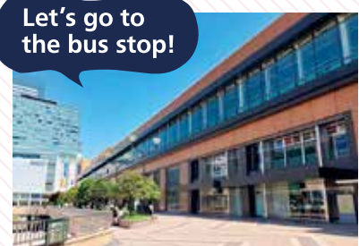
This is the West Exit Pedestrian Deck on the 2nd floor of Sendai Station.
